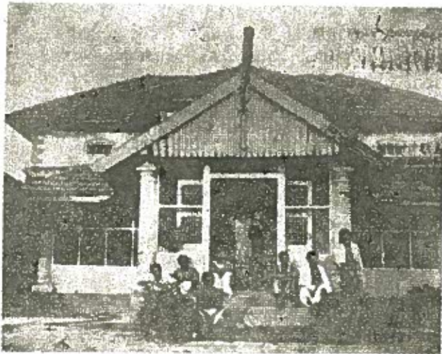
Govt. Hospital, Kattoor
